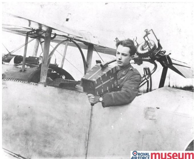
Figure 16: Lieutenant S C Thynne demonstrating the use of a Thornton-Pickard Model 'A' handheld camera from the back seat of a Nieuport aircraft.
