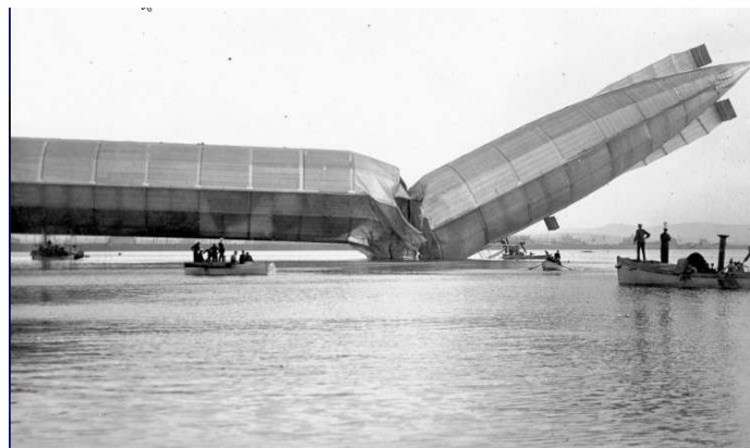
Figure 2: HM Airship No.1 'Mayfly' broken in half after strong winds hit the side of the airship. It was also believed that one of the mooring lines had not been released and that the airship was literally pulled in half. Images from the collection of Vice Admiral Sir Cecil Ponsonby Talbot.
